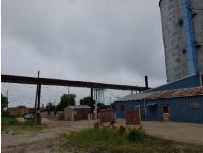
114. Outside large generator room
