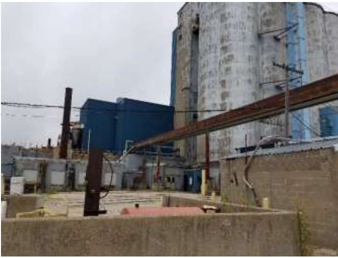
1. Overhead transmission line
