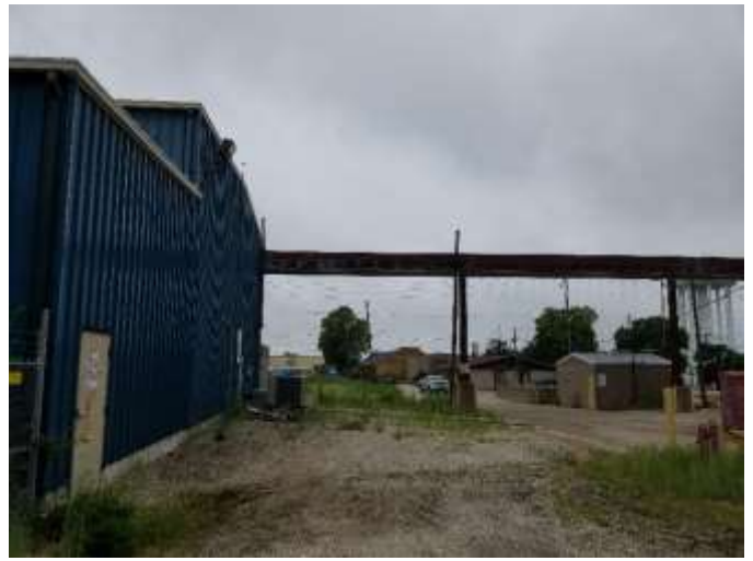
113. Outside large generator room
