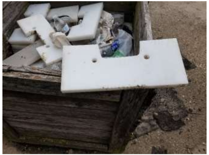
78. Parts inside building #2
