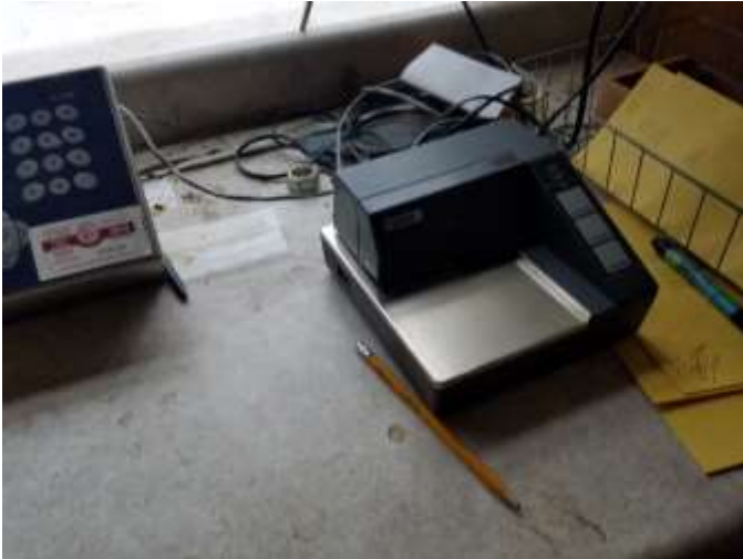
88. 90 foot truck scale equipment
