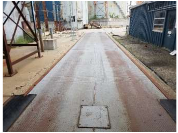
87. 90 foot truck scale equipment
