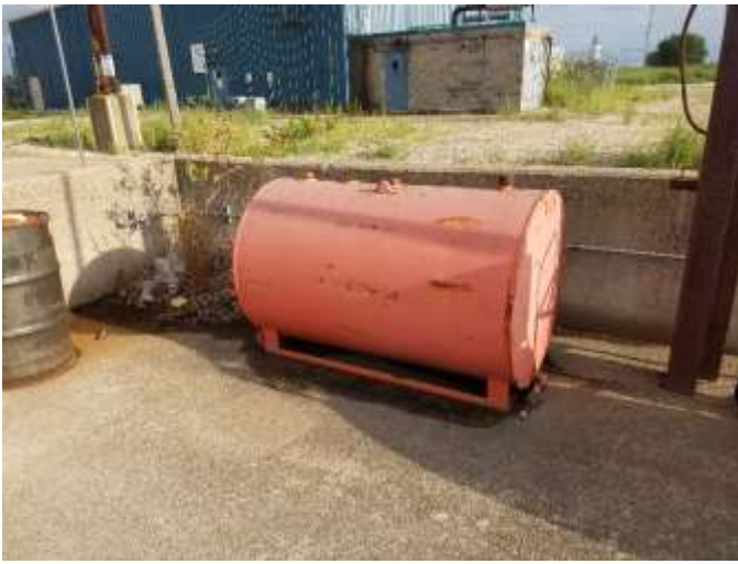
195. Red 500 gallon tank used oil
