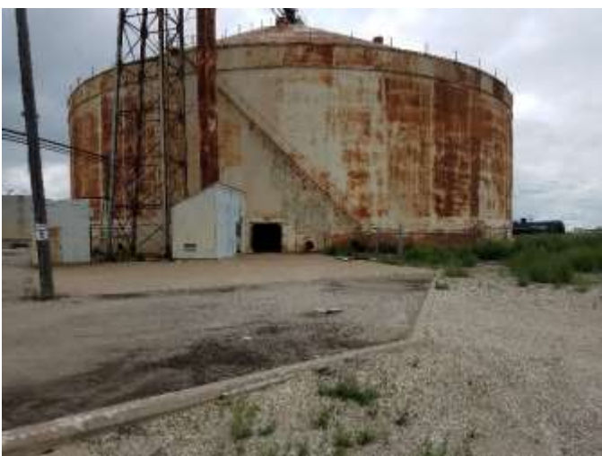
7. 1.5 million bushel steel grain bin with top & bottom augers
