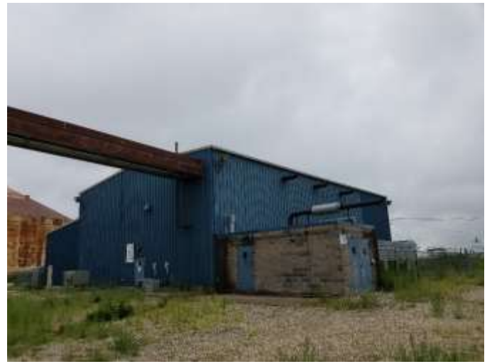
2. Overhead transmission line
