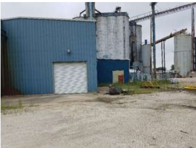
126. Outside of generator room
