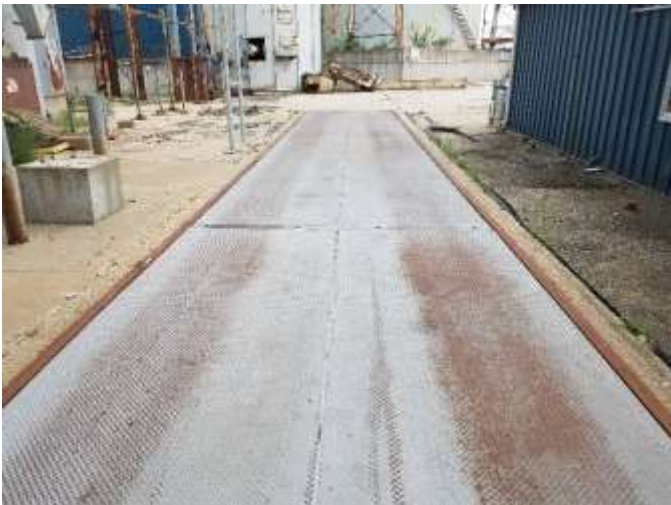
90. 90 foot truck scale equipment
