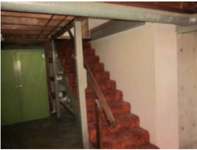
Stairs to basement
