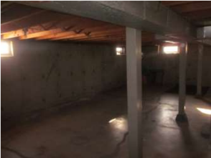
Front half unfinished basement
